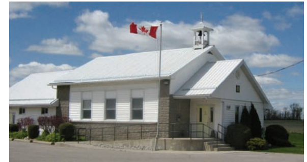
Lions Community Centre County Rd 10 at Larmer Line, Millbrook
